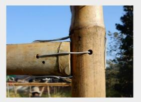
Side joints between bottom chord and side column.
