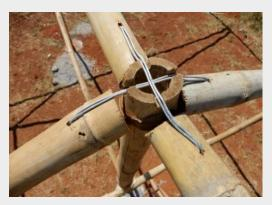
Joints between the center column, rafter, and purlin
