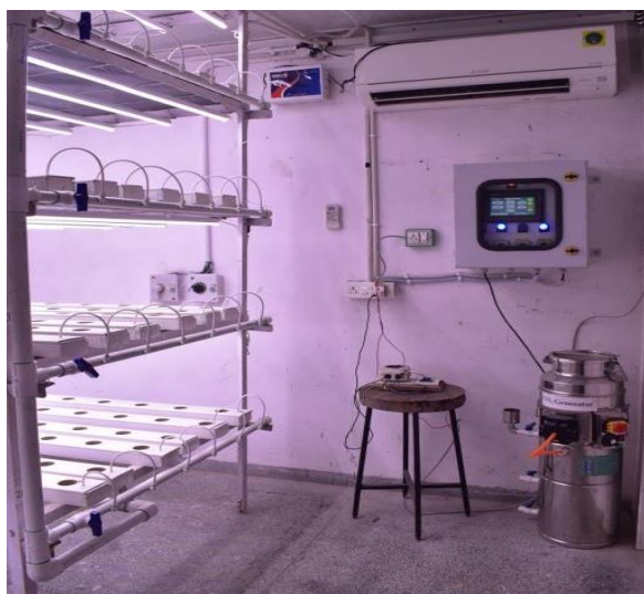
Air Conditioner, CO 2 generator and Humidifier connected with PLC control panel
