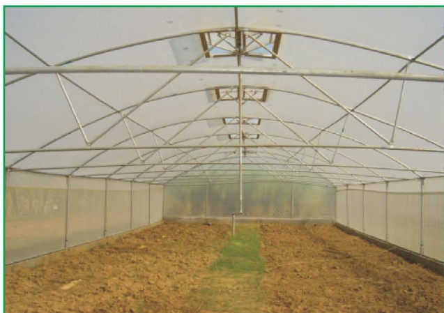
Modified naturally ventilated polyhouse
