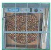
Desiccant wheel fitted on the evaporative cooler
